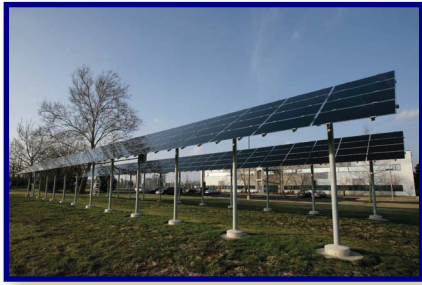
Figure 7: Array of thin-film photovoltaic panels powering an entire building at the University of Toledo campus, Toledo, Ohio, USA.
